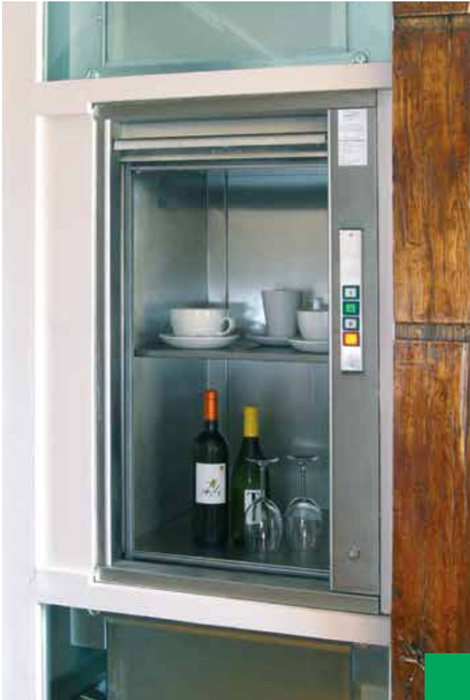
Installation in a restaurant (UK), model 50 kg, with glass cladding.
